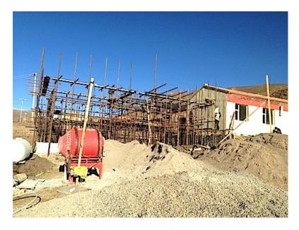
Very solid steel reinforcements to make the canteen safe, in case of an earthquake, though Huanquhu has no records of earthquakes.
