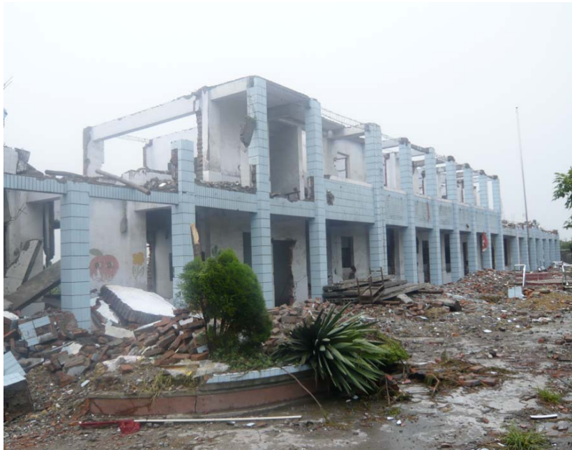
Post-Earthquake School Campus, July 29, 2008
